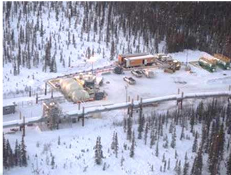
Slip Stream Heat Operation
