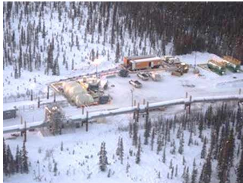
Slip Stream Heat Operation
